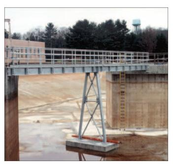
Design and fabrication performed in-house. Hot-dip galvanized steel, weathering steel or painted applications.
